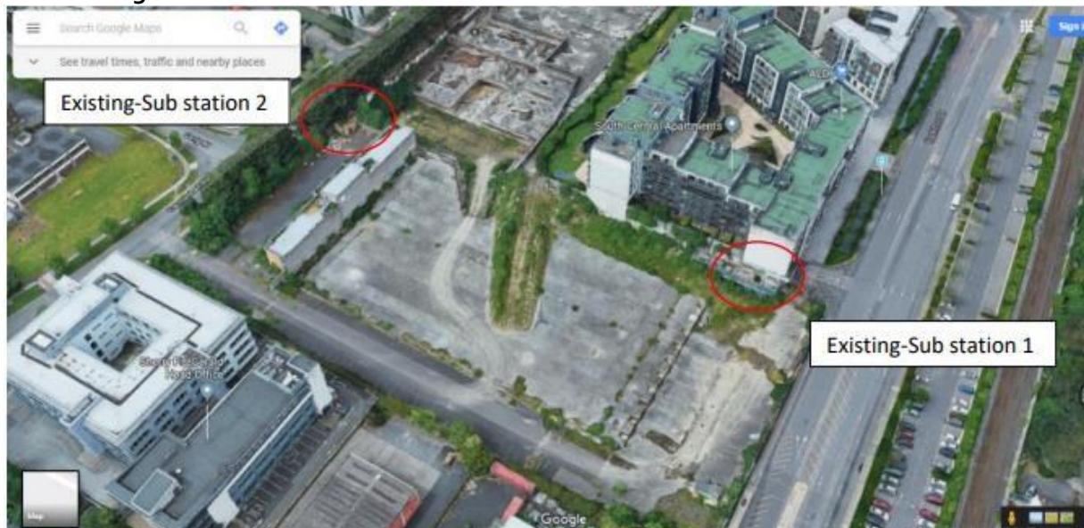
Figure 17.7: Existing Substations on Proposed New Site.
